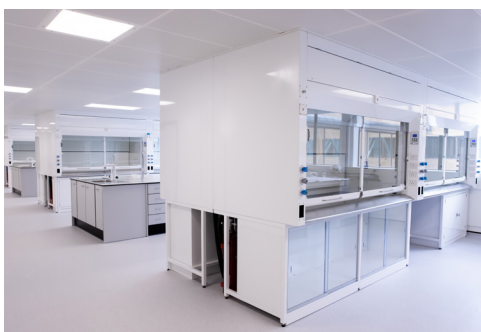
Banks of fixed fume cupboards
