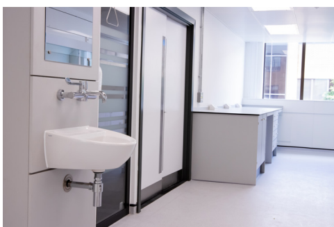
IPS unit & fixed underbench storage
