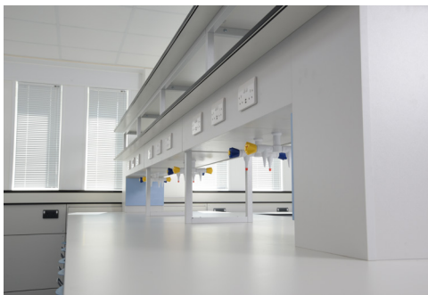
Reagent shelving /gas outlets & twin USB sockets
