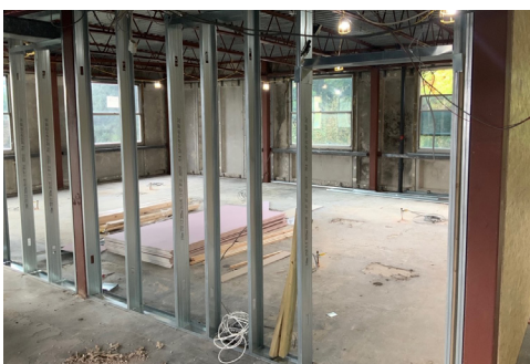
Work in progress - rebuilding partition walls
