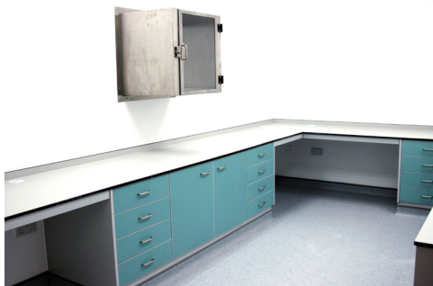
Access hatch to adjacent laboratory
