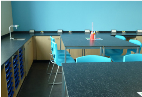
Trespa benching with perimeter services
