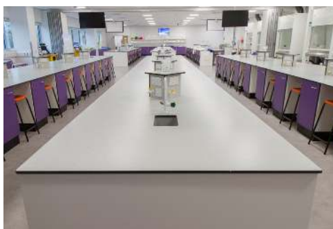
Practical laboratory with raised service turrets
