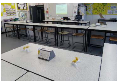
1200 x 600mm Trespa service bollard
