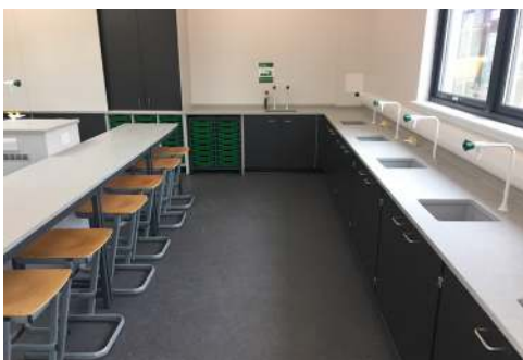
Perimeter benching with 25mm Velstone worktops
