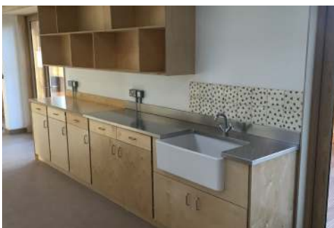
Stainless steel bonded onto MR MDF substrate
