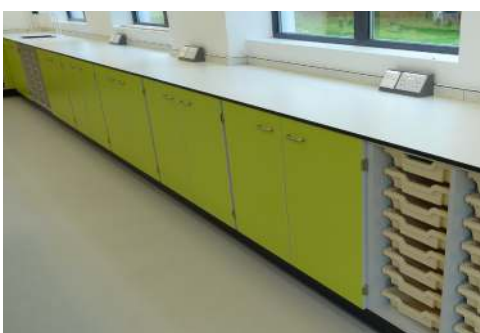
Perimeter Trespa benching with lime doors.
